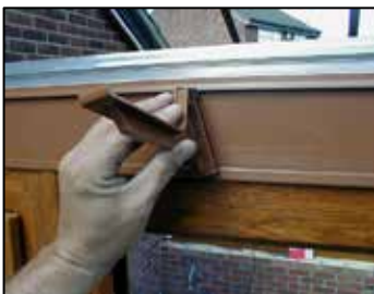
1) Gutter Brackets must be fitted at a maximum of 600mm centres and no more than 200mm from each corner. The Gutter Brackets are located in the Ring Beam External Trim and are twisted into position as shown.
