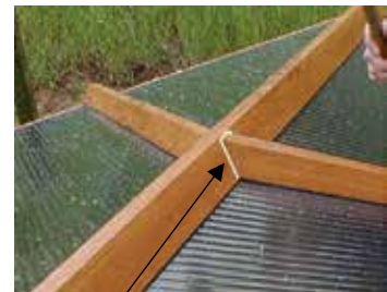
2) Place the Jack Rafter into position, locating the Jack Rafter Bar onto the Jack Rafter Fixing and onto the Double Studs at the Ring Beam End. Tighten all nuts.
