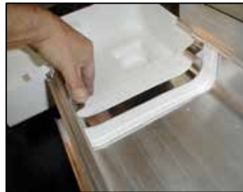
5) To fit the other section of the Box Gutter Brace, lower it into position and then apply pressure in the position shown to cause compression to enable the brace to be clipped into position.
