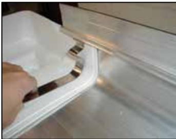
4) Position the Box Gutter Brace in the Groove on the adaptor with one part of the Brace hooked into position.
