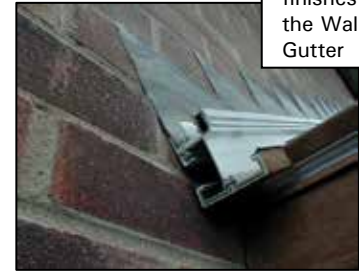
Mitred Eaves Beam Seal
