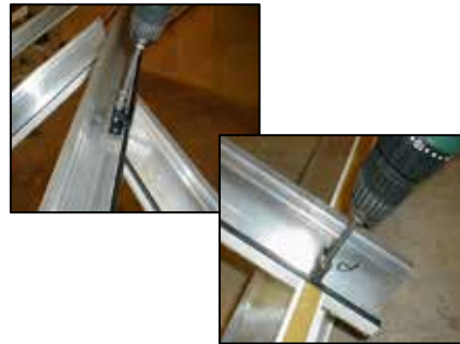
2) Place the Jack Rafter into position, locating the Jack Rafter Bar onto the Jack Rafter Fixing and onto the Double Studs at the Ring Beam End. Tighten all nuts.
